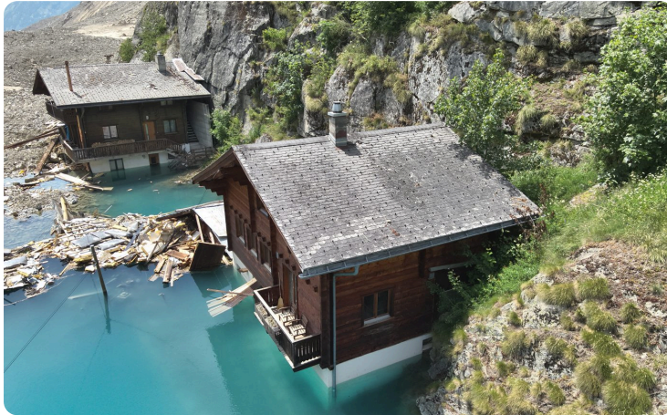
Drone image of June 2025: chalets standing in the lake dammed up by the debris.
