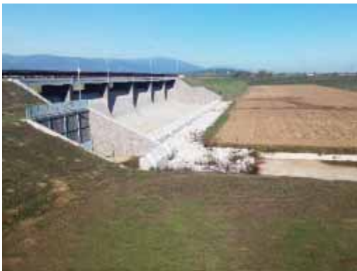
Dry reservoir used for temporary water storage to reduce the risk of flooding the towns downstream. The 110 hectares of the reservoir are also used for farming (Italy)
